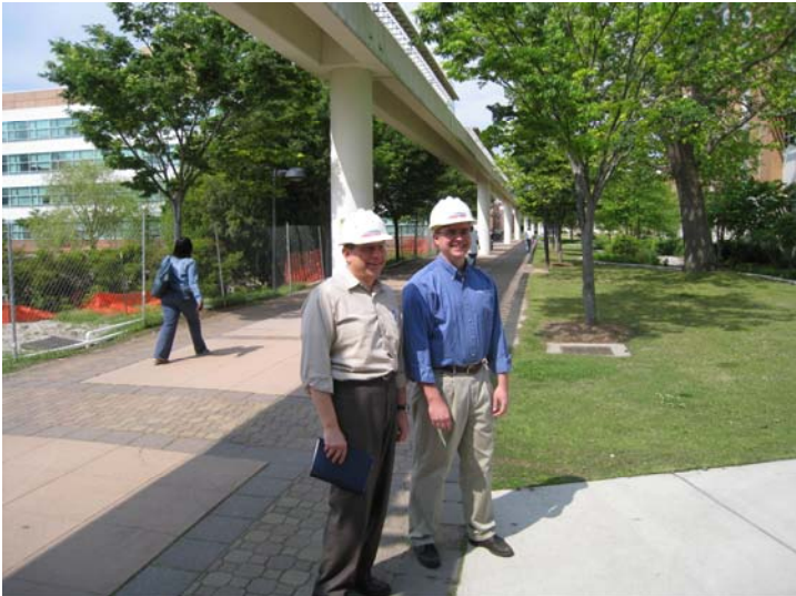
Fig. 1. Section of existing maglev guideway at ODU.
